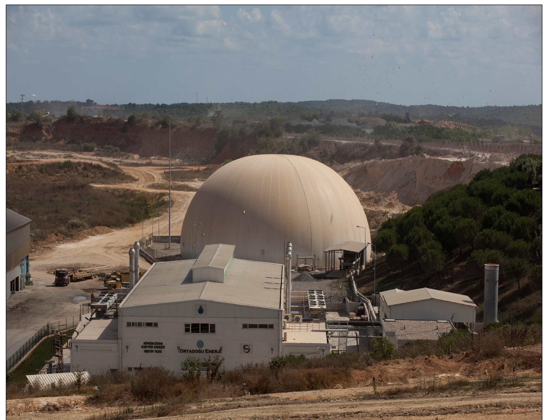
LFG Energy Plant
