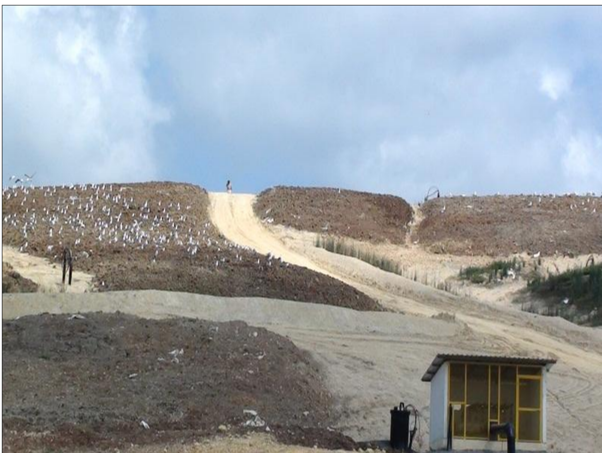
Closed Portion of the Landfill
