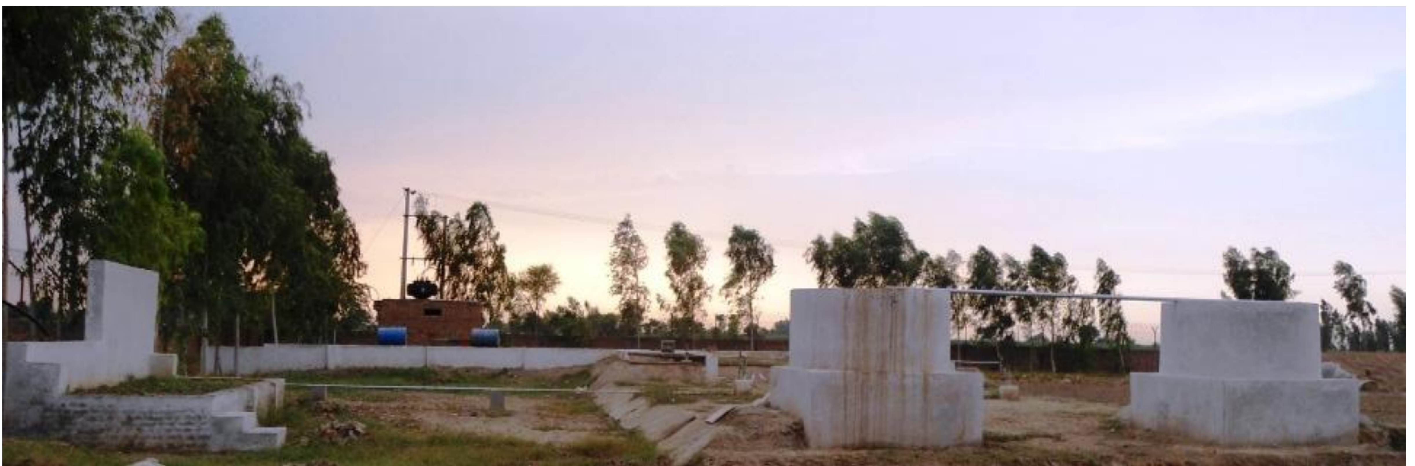
Biogas Plant at Nestle' Farm
