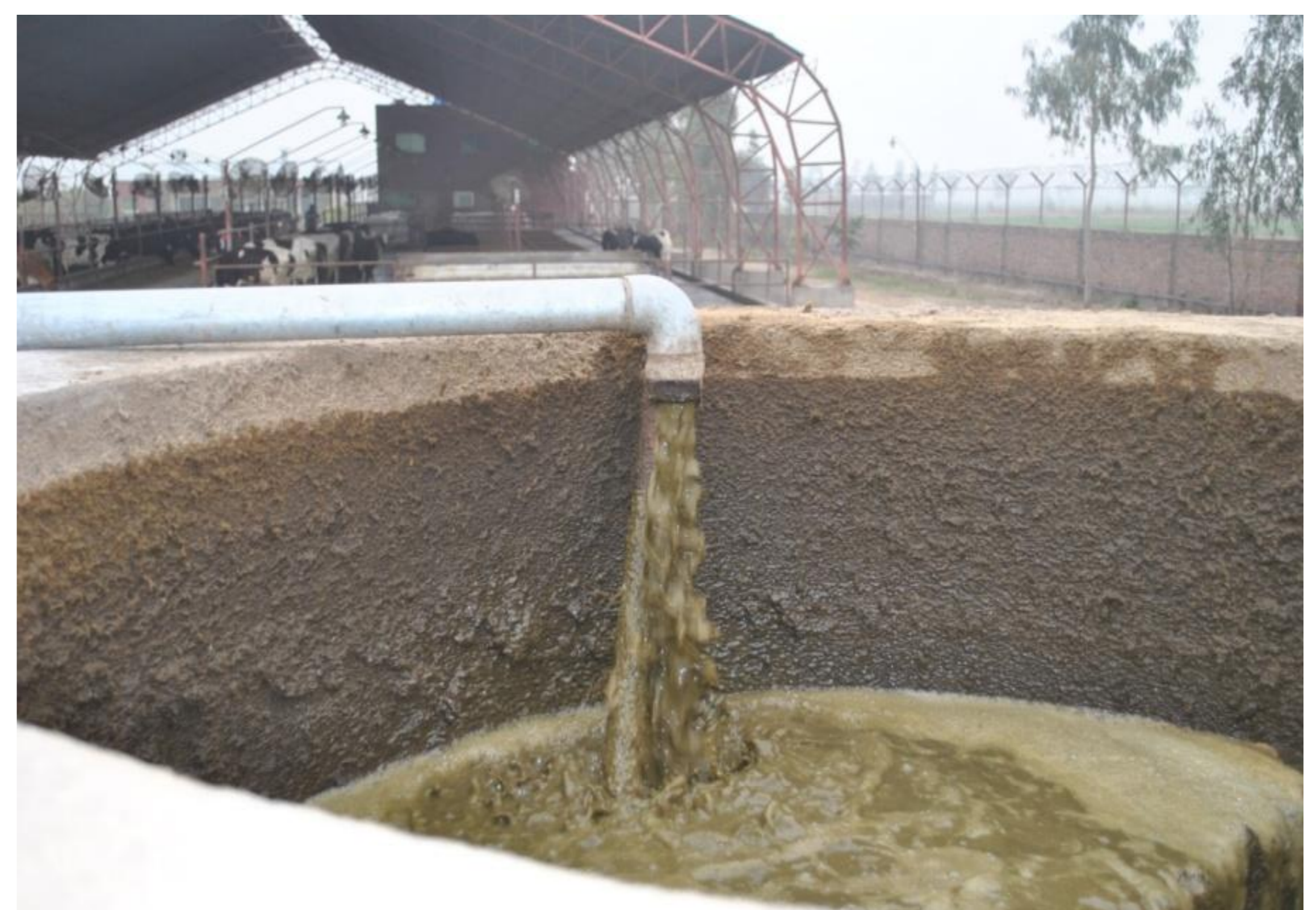
Inlet being filled with Manure-Water Mixture
