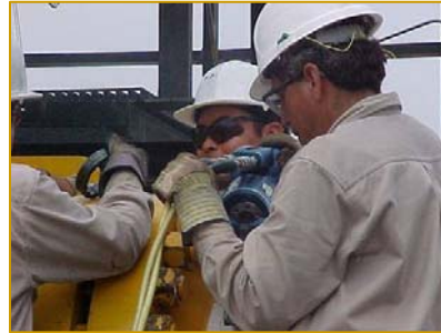
Tightening with Hy-tork Equipment
