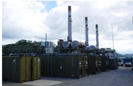
1 bio-gas generator of Fudekeng provides 1.361MW
