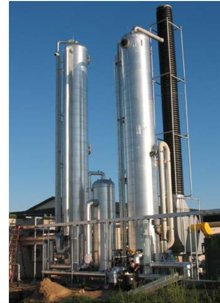
Fair Oaks, Indiana Totara+ System Installation
