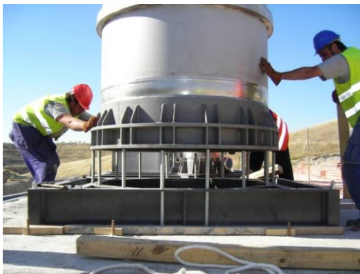
Greenlane® Totara – Scrubber Vessel Installation
