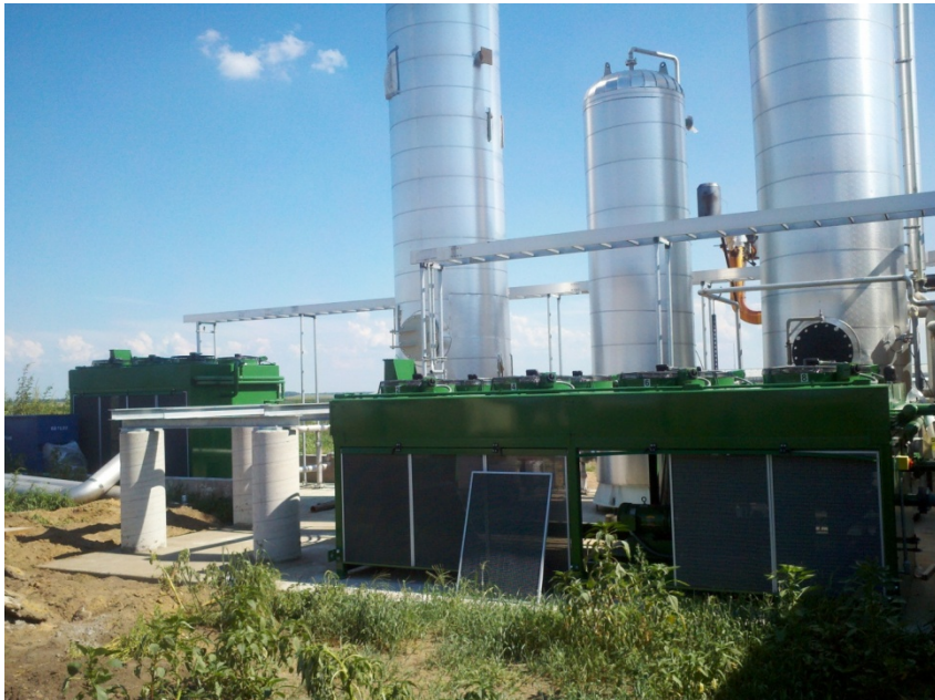
Gas Cooling and Water Chilling
