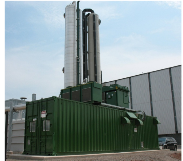
City of Hamilton, Ontario 'Rimu' System Installation
