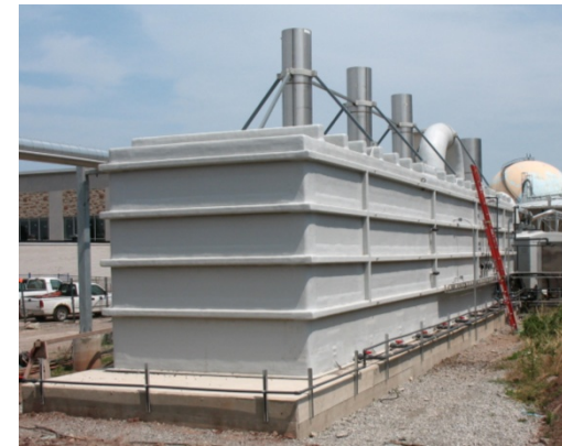
Biotrickling Filter
