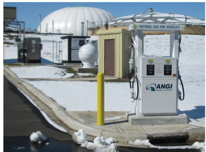
Wastewater biogas to CNG vehicle fuel project, Janesville WWTP (Janesville, Wisconsin, USA)
