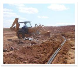
Figure 4-1. Installing a HDPE LFG pipeline for the Brazil MARCA Landfill in Cariacica, Brazil
