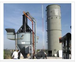
Figure 4-5. Leachate Evaporator System at El Verde Landfill in León, Mexico
