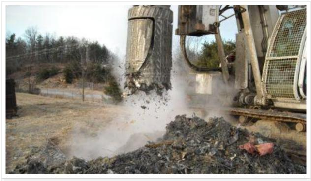
Figure 3-5. Vertical Extraction Well Drilling
