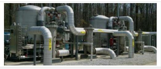
Figure 4-11. Siloxane removal systems at the Lorraine power station at Oberlin, Ohio, USA
