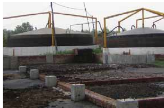
Floating dome anaerobic digestion of animal wastes in India.
