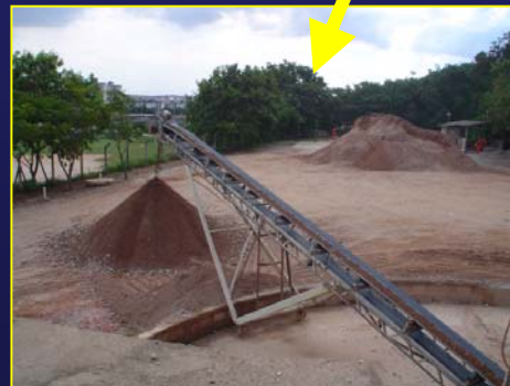
Construction Waste Recycling
