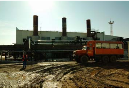
Installing 45 MW Gas Turbine in Saly
