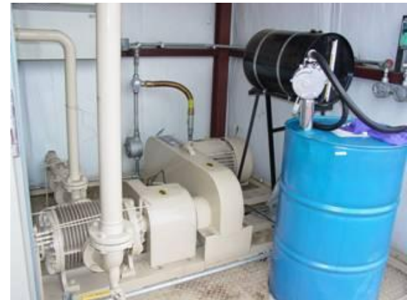
Baker, MT ConocoPhillips VRU installation Pictures Courtesy of Hy-Bon Engineering
