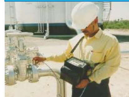
Acoustic Leak Detection
