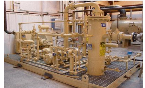
Baker, MT ConocoPhillips VRU installation Pictures Courtesy of Hy-Bon Engineering
