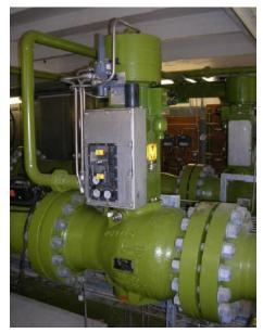
Axial Style Valve Equipped with Moore 750 pneumatic positioner, two inch (50mm) diameter piping used to vent gas to atmosphere
