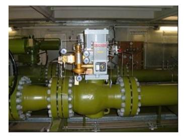
Becker High Pressure Positioner (HPP) and LPDA actuator allows gas to be discharged into a downstream Bleed to Pressure system eliminating ALL emissions
