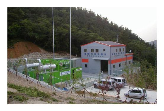
No. of units and engine type: 2 x JGC 320 GS-L.L
