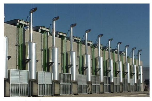
No. of units and engine type:  $11 \times JMS 420 GS-L.L$
