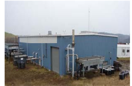
Photos courtesy of Montauk Energy
