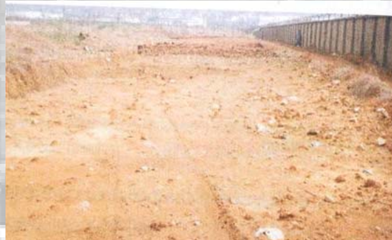
After Shifting and Capping
