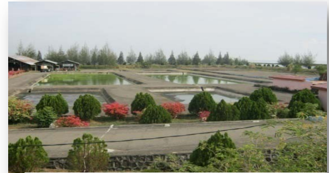
Septage treatment plant
