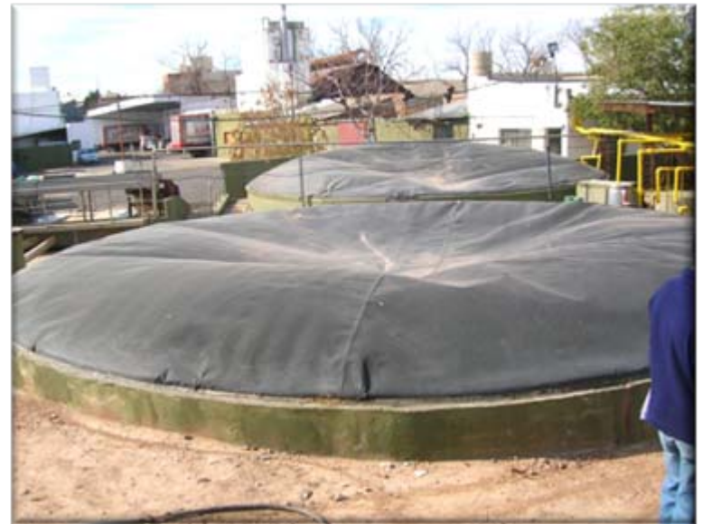
Sugarosa Rosario Santa Fe province slaughterhouse operation 4 digesters green line 1800 m 3 capacity covers 32 % of energy needs 132.000 m 3 per year 1998 – 2001 in operation
