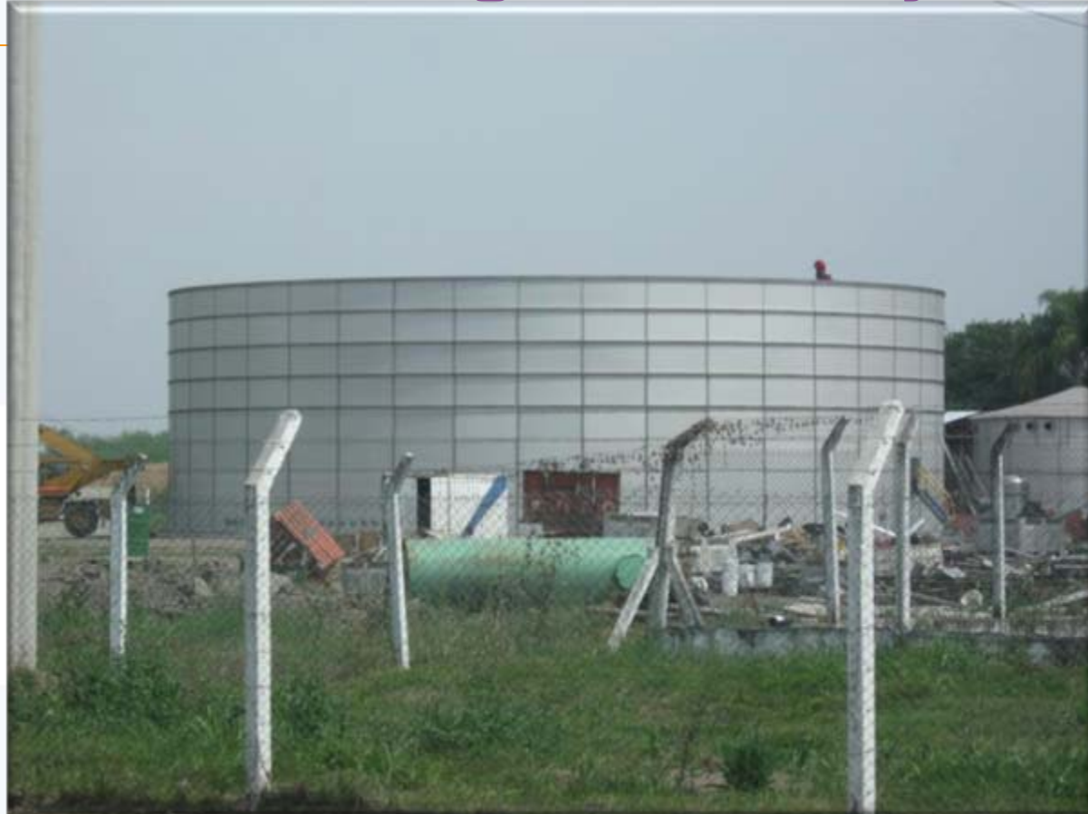
Citricola San Miguel New 7000 m 3 UASB type digester on citrus agro industry Tucuman province initial load February 2009 - 2010
