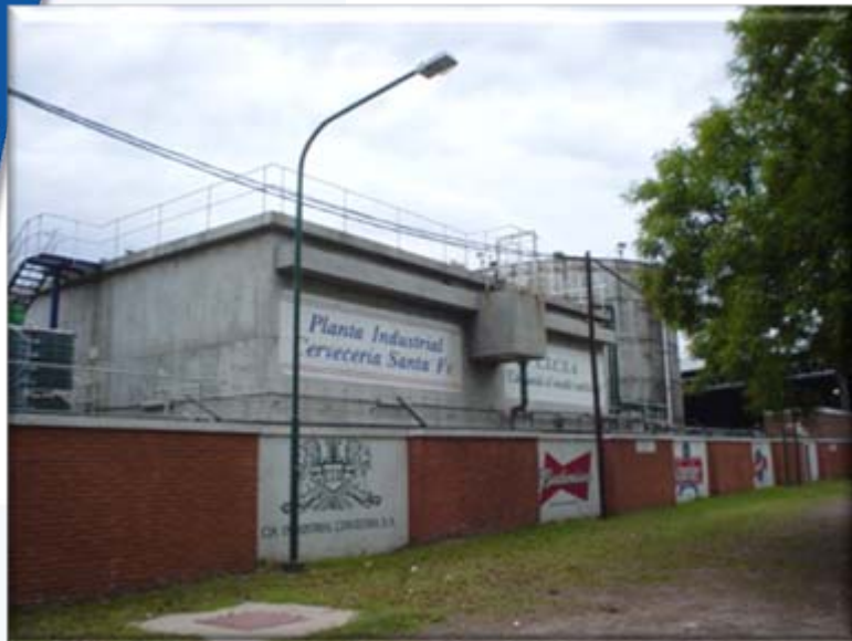
AD in Brewery Santa Fe province 2400 m 3 Production 1 million m 3 biogas per year used in the factory in operation since 2001
