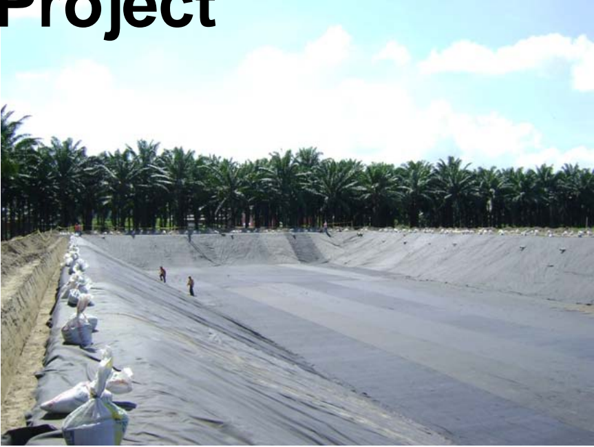
Geotextile Installation
