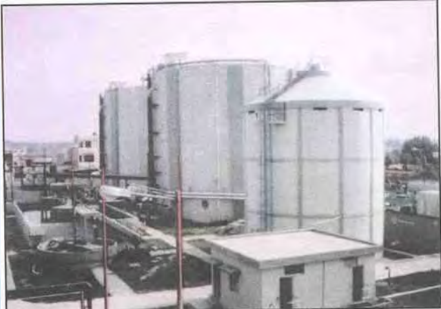
Two BIMA Digesters and the Gas Holder
