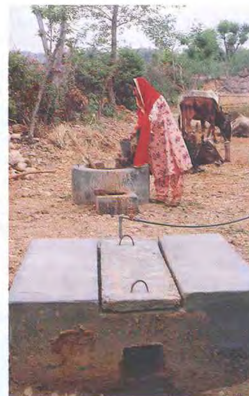
A Deenabandhu Biogas Plant at Deoli Village, Himachal Pradesh.
