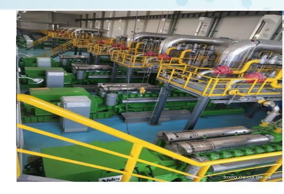
New CMM power project with total capacity of 30MW, using GE Jenbacher gas engines at Shihao Coal Mine of Chongqing City.
