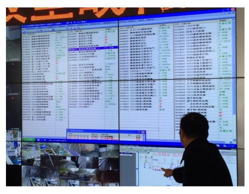
Figure 2-5: Screen Providing Real-Time Feedback on CH<sub>4</sub> percent, Air Velocity, Etc.
