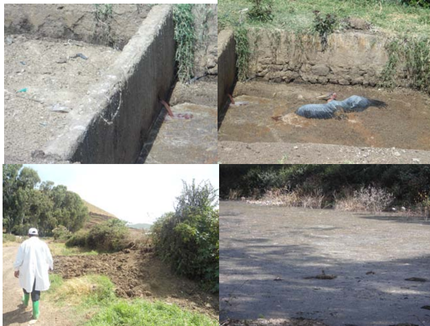
Waste disposal system of ELFORA Abattoiri in DebreZiet. Pond, man-made lake, and solid waste pile
