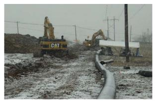
Pipeline installation for direct-use project at Conestoga Landfill, PA
