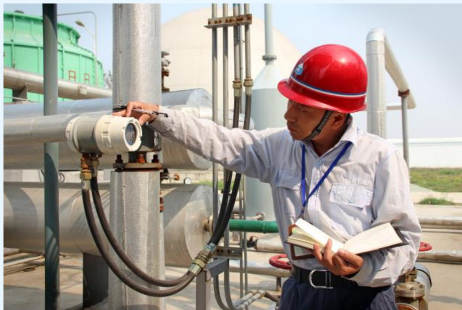
The Xiangyang sludge-to-energy plant, used with permission courtesy of TOVEN.
